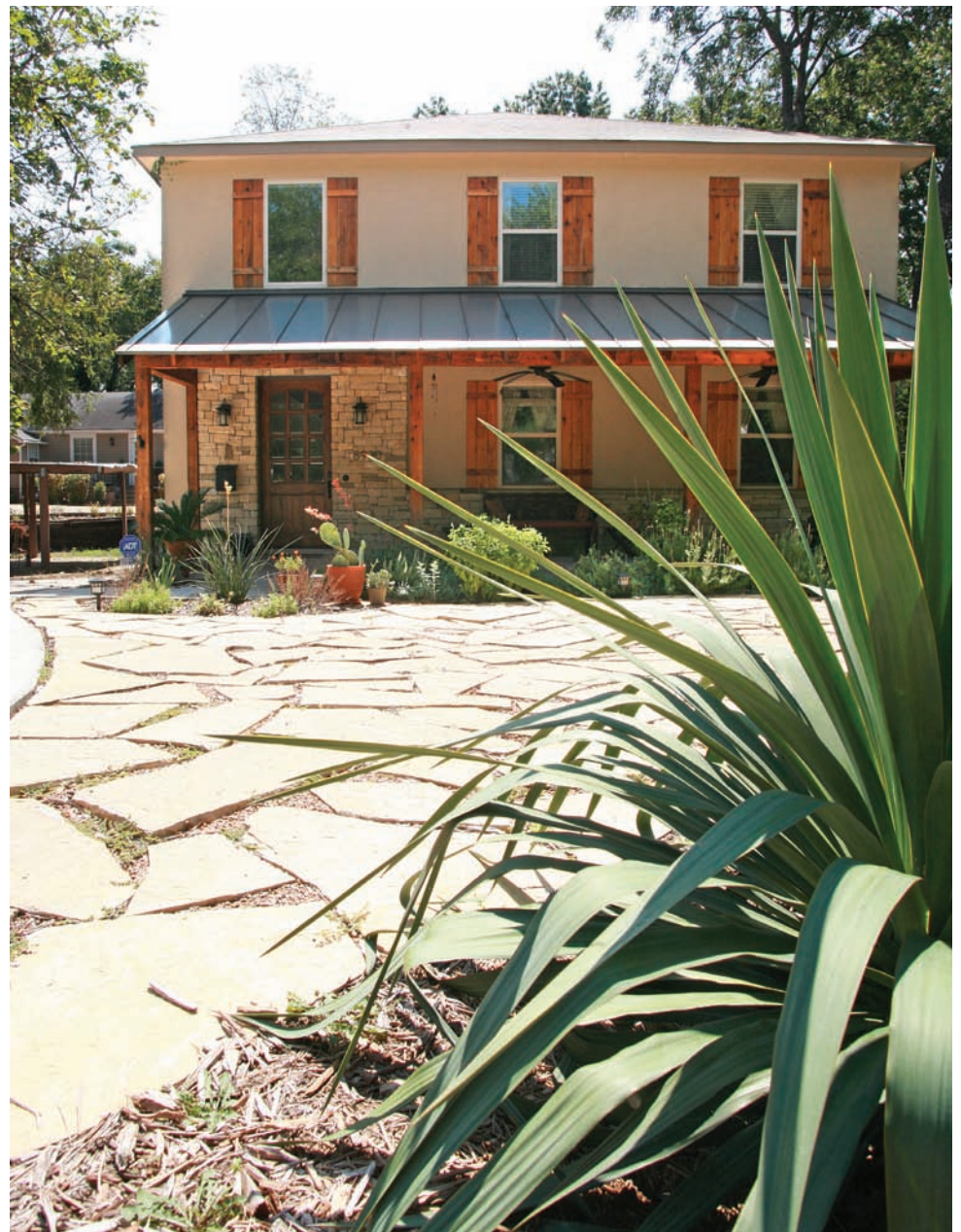
With its xeriscaped yard, metal roof covers, and Western cedar flank shutters, the exterior of Anna Clark’s home sets the tone immediately for a LEED certified house.
